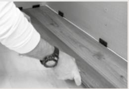
Start from the left corner of the room, having the tongue clinging to the wall, foreseeing to leave a perimetral space at least 8 mm, using spacers (do not fill with silicone, wires, etc.).
