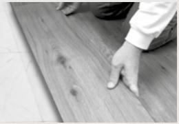
Fix using the tongue-and-groove method.
