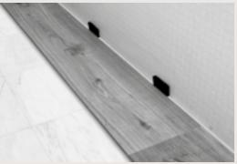
Leave a distance of 8 mm on the entire room perimeter and from every obstacle that could compromise the laying movement. Once the laying is completed, remove all spacers and place proper skirting board. Do not fix the skirting board on the floor.
